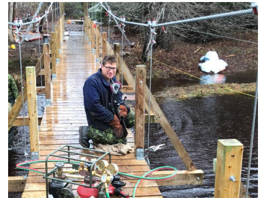
Cfn Szustakowski (OJT) involved in the suspension bridge construction in Ingonish (2017).
